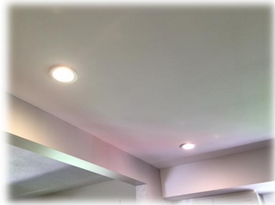
Recessed task lighting used over counters
